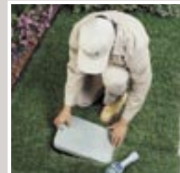
Replace the valve box cover and the hermetically-sealed WVC is protected from water, dirt, and contaminants.
